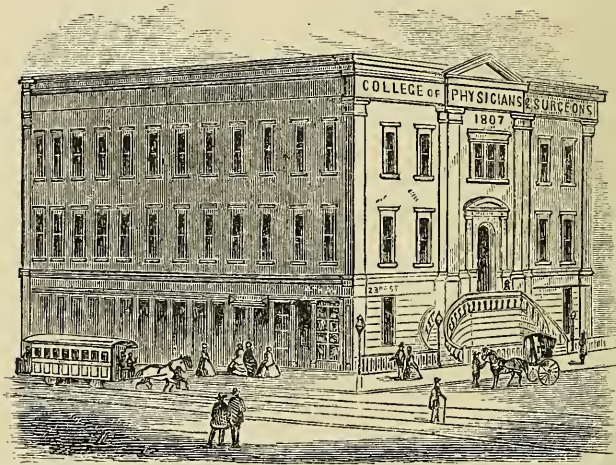
THE COLLEGE BUILDING IN TWENTY-THIRD STREET.
